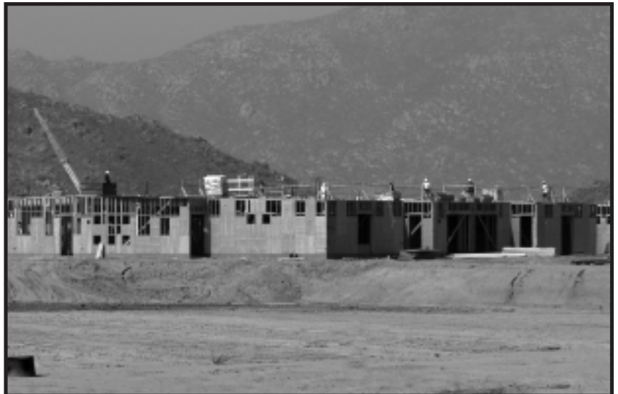
Tahquitz High School Construction
